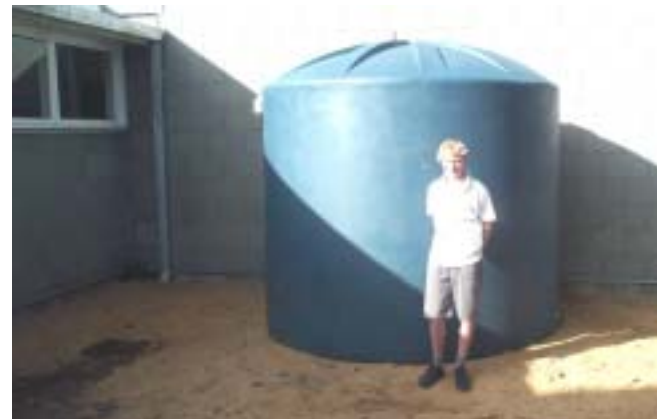
Above: Ben checks out the new drinking water tank.
